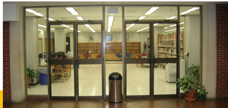
Renovations of the garden level of Moody Memorial Library are scheduled to begin this summer.
